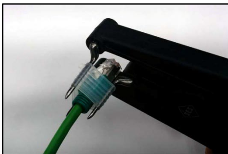
FIGURE 10 - INSERTING RJ-45 END THROUGH SHROUD
